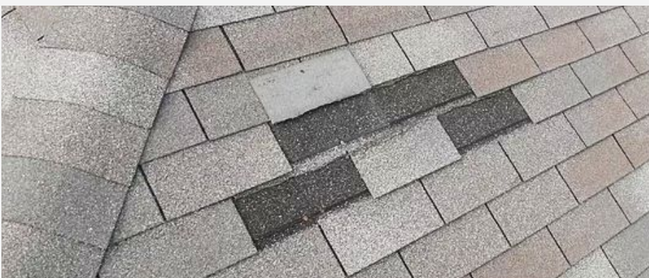
MISSING SHINGLES
